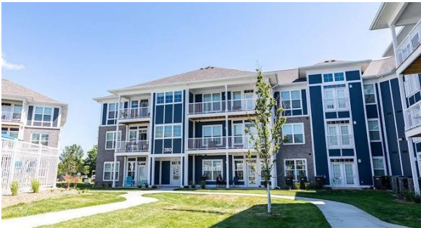
Elevation Apartment Homes Alexandria (Campbell) · 327 units · 2023
